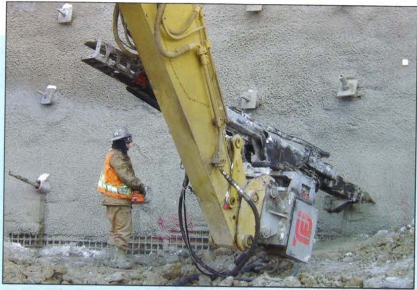
Figure 6: Excavator-mounted TEI Drill.
