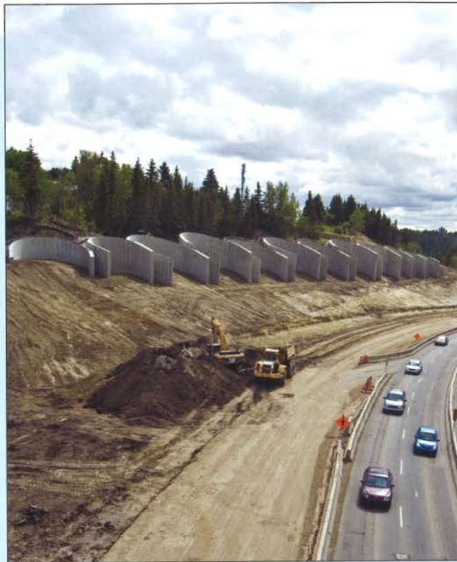
The completed shoring wall adjacent to Whitemud Drive.
