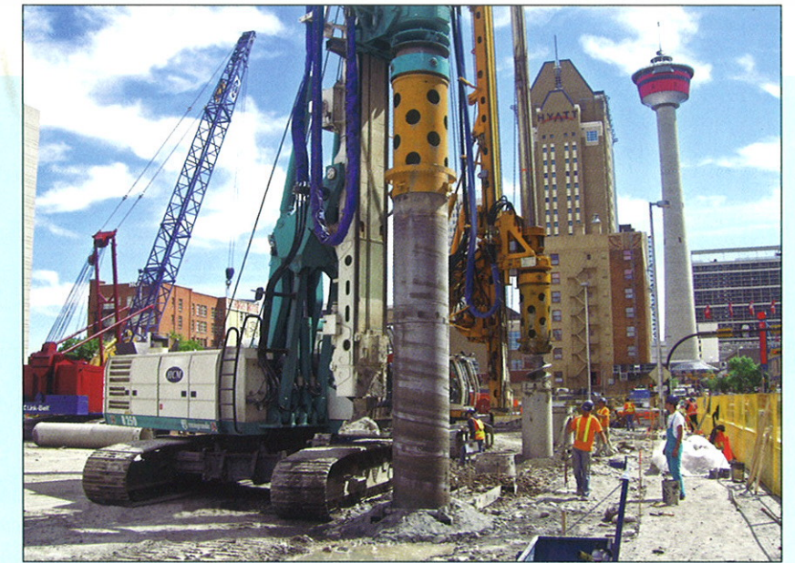
Casagrande B250 and Bauer BH-24H drilling first sequence of secant wall.
