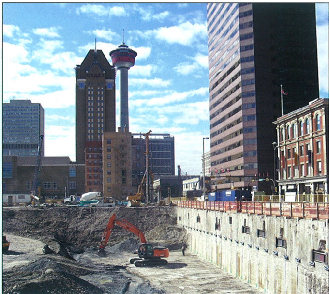
West wall trimmed and ready for second row anchor installation.
