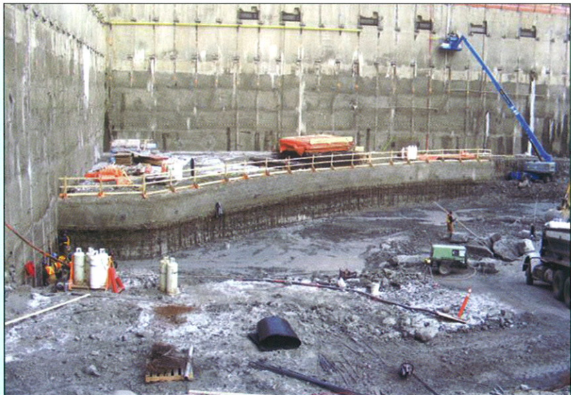
Raft slab construction using shotcrete shoring.
