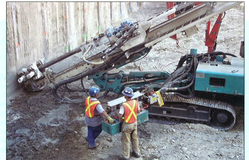
Casagrande M9 drilling for top row anchors in secant wall.
