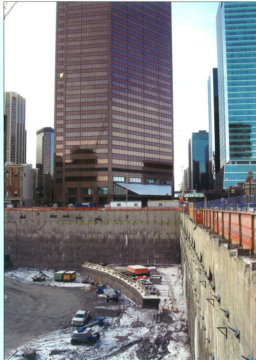
Northwest corner of the site where special shoring was constructed for forming of The Bow raft slab on grade.
