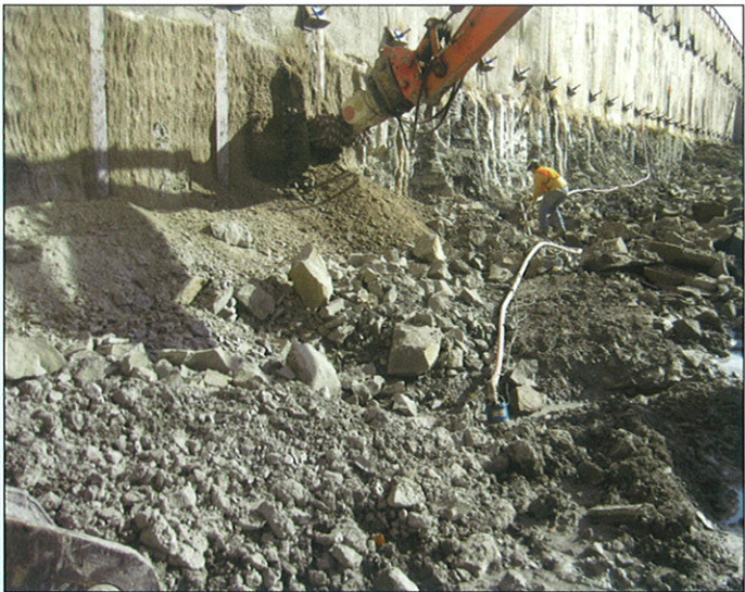
HCM rotary cutter trimming secant wall flush and preparing transition to shotcrete.
