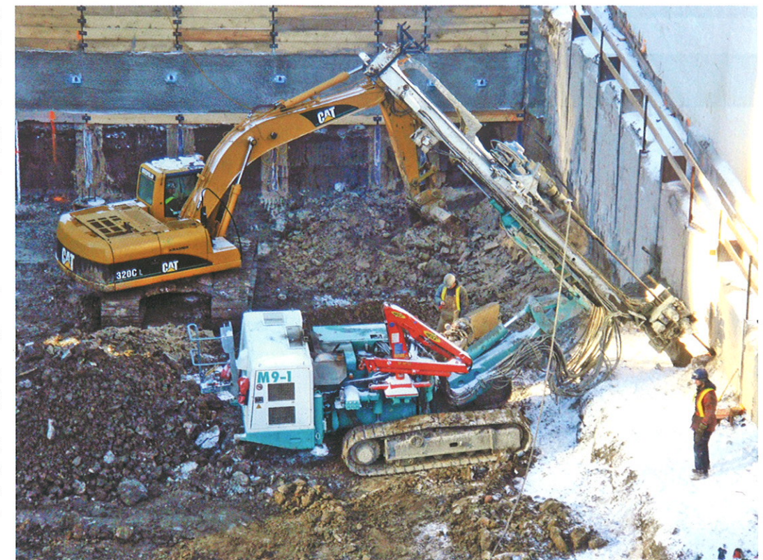
Figure 1: Installing high capacity tiebacks on north wall.
